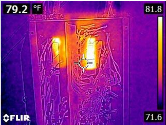
9.2 Item 4(Picture) Distribution panel infrared
