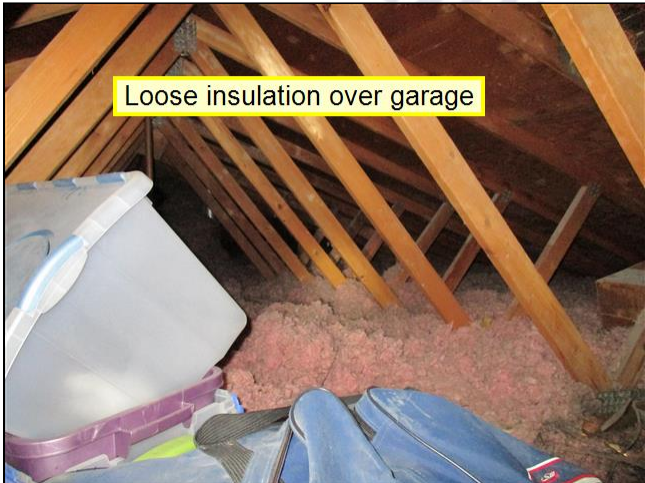
1.6 Item 1(Picture) Insulation over garage
