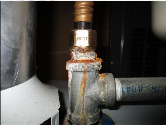
8.1 Item 2(Picture) Corrasion on water heater
